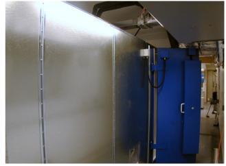
The beam end of the Faraday cage (top left), soon to be covered by a shielding wall, the side entrance (top right) and the cage ceiling, showing how ventilation ducts and three-phase power input cables interface to the cage. The power is filtered with custom RFI filters (C, L, C 'PI') on all lines.
