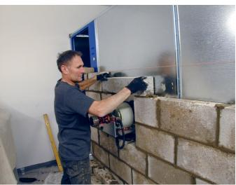
Covering the beam line end of the Faraday cage with staggered, offset blocks.
